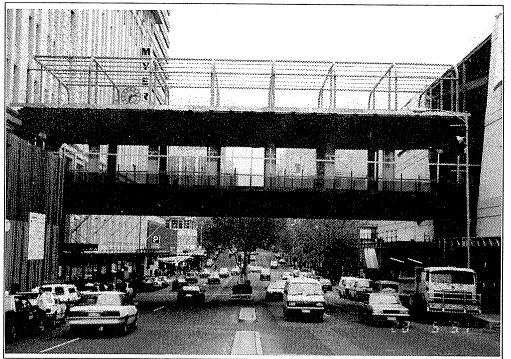
▲ The bridge under construction
