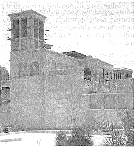
▲ Traditional wind tower
