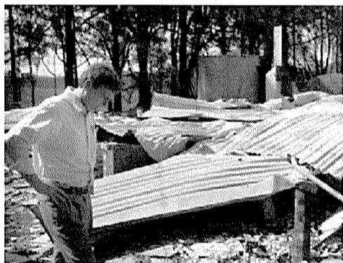
▲ Former Victorian Premier, Hon John Brumby inspects the destroyed Callignee Hall
